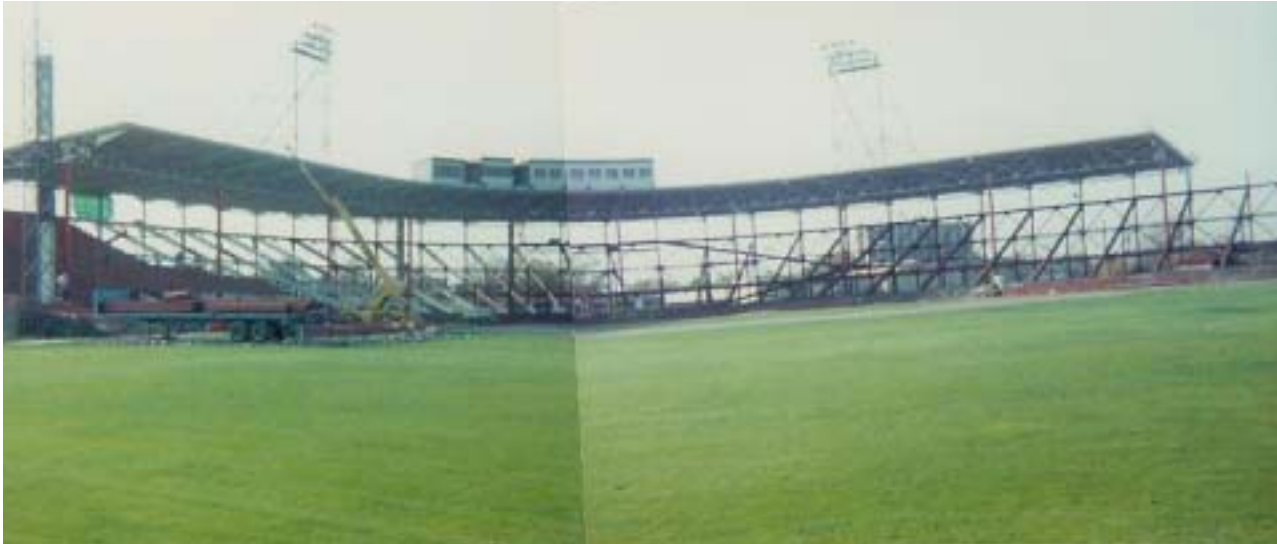
Silver Stadium during the refurbishing, 1986 (photo by John Walter, RochesterAreaBallparks.com)
